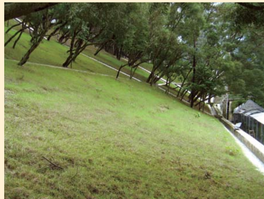
在邵逸夫人樓附近的回填坡，是藉挖坑種植來鞏固的。這種方法可盡量減少移植樹木，部分過程須用人手處理，耗時較長。 A more time-consuming method of stabilization—trench excavation—was used to stabilize this fill-slope near the Lady Shaw Building so tree removal can be minimized. Part of the procedure was carried out manually.
