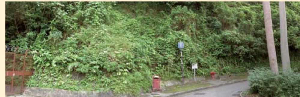
九十年代在崇基職員宿舍附近蓋滿灰泥護面的斜坡（上圖）；同一斜坡的現貌（下圖）。 Before: a slope covered with chunam plaster near Chung Chi staff quarters in the 1990s (top) After: the same slope now (above)
