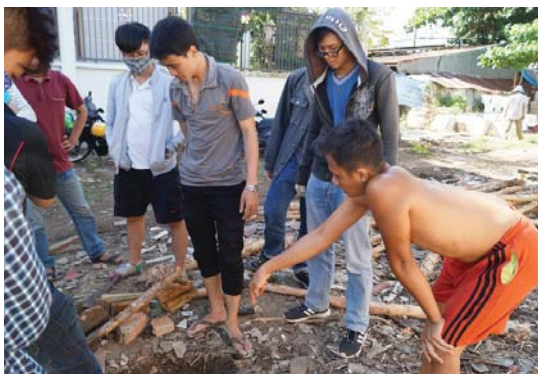
A resident offers some advice on putting the X-shaped posts into the ground
