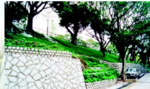
Trees and Shrubs are planted on the slope.
