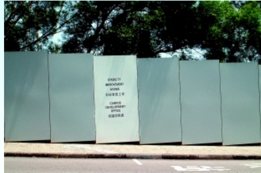
Hording of Construction Site
