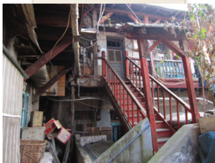
里院院子裡的樓梯 Staircase inside Liyuan courtyard
