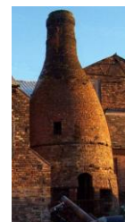
燒陶器的 Bottle Kiln（右側的已成為博物館展品） A bottle kiln for firing pottery (the one on the right has been preserved as a museum exhibit)
