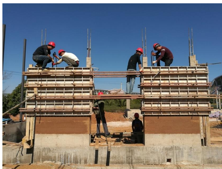
Figure 11. Rammed earth wall construction of the Terra Centre.
