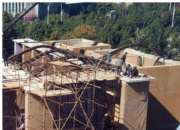
Figure 13. Construction of bamboo roof structure of the Terra Centre.
