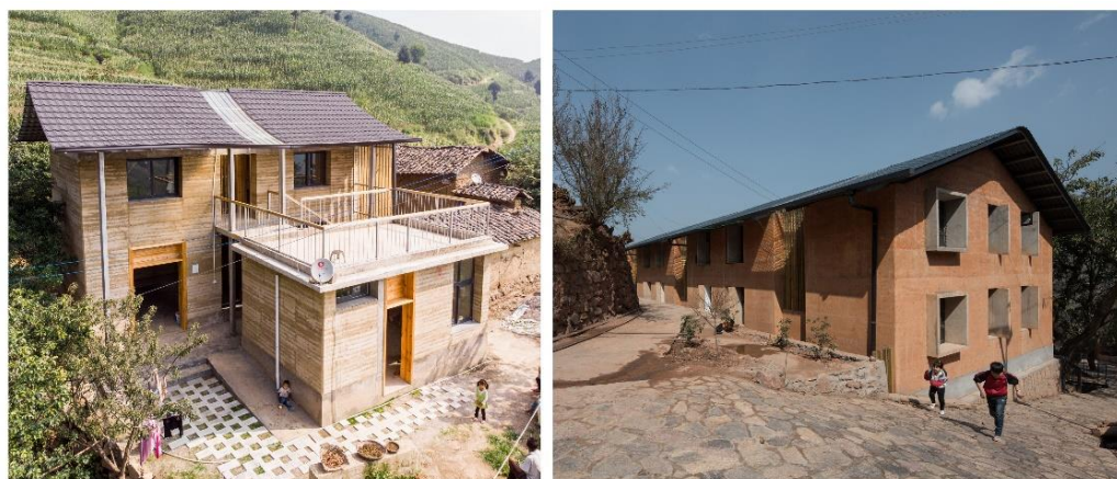
Figure 18. New rammed earth houses in Sichuan and Yunnan built by the villagers' construction team, with the support of the Terra Centre.
