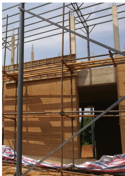
Figure 12. Concrete tie columns and ring beams of the Terra Centre.
