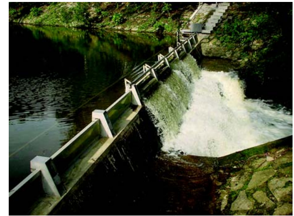
The automatic watergate installed in Wei Yuen Lake is made of stainless steel and reinforced glass with four vents. The water level is adjusted by the sensor.
