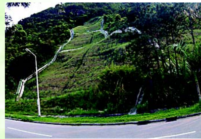
A steep slope has now been made more gentle and fixed by 1,000 soil nails, hydro-seeded and covered with an erosion control mat. 原本陡峭的斜坡，現已變為緩坡，固以千枚泥釘，草種和水敷播，並覆上保護蓆，防止土壤流失。
